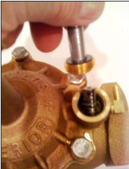
**6.** Photo of solenoid cavity. The o-ring seal can be seen at bottom of cavity. The port in the center of the cavity is the exhaust port. The other port connects the diaphragm chamber to the solenoid chamber.
